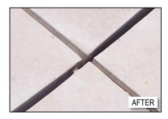
Climatic conditions must be taken into consideration before the repair is to commence. Do not repair stone in freezing weather or if a freeze is anticipated within 24 hours. On hot sunny days repairs should be done during the morning hours where the cast stone is shaded or at temperatures less than 90 degrees Fahrenheit. Repairs should be covered with a damp cloth and plastic sheet to prevent the water from evaporating before the cement has hydrated.
