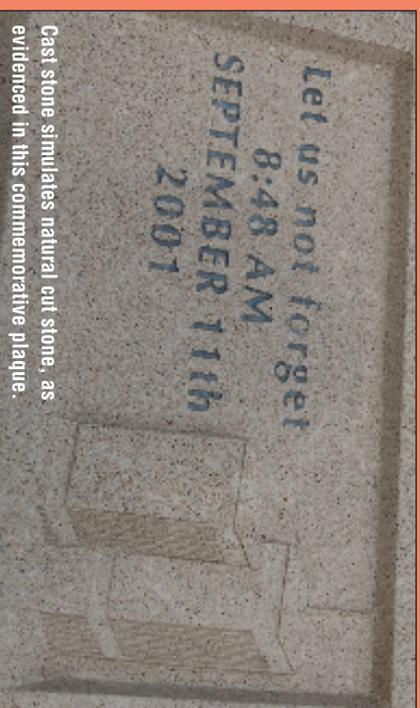
Cast stone simulates natural cut stone, as evidenced in this commemorative plaque.
